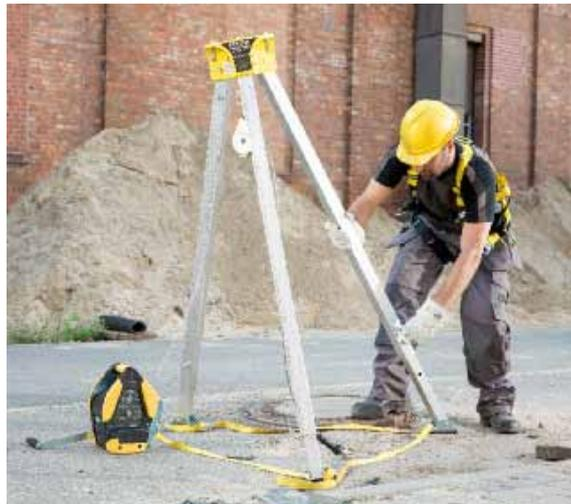
task-specific work (such as manhole entry), are easily transported and can be set up by one person.
