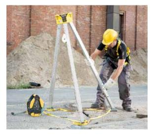
presence of harmful fumes, creating a need for a fall arrest lanyard or device which stops a fall in progress.
